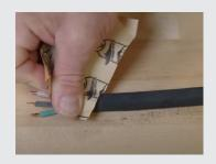
**5** SWAB or clean the wires, sheathing, internal disconnect body and end nut thoroughly with alcohol or alcohol wipes to remove any debris and allow them to dry completely.
